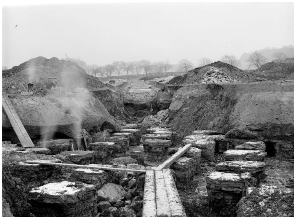
Room and pillar workings discovered in foundation excavations for Cowglen Hospital, Glasgow, 1937
