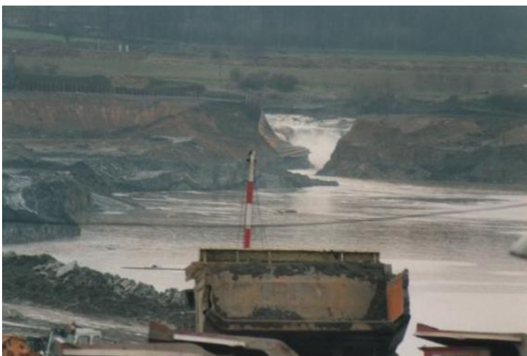
1988 St Aidan’s Extension Opencast Mine. The sidewall collapse brought the River Aire and the Aire and Calder Canal into the mine workings. In spite of downplaying its significance this collapse, which cost many tens of millions of pounds, altered geotechnical practice in surface mining and quarrying across Britain and led to changes in the law. Similar large collapses have taken place subsequently.
