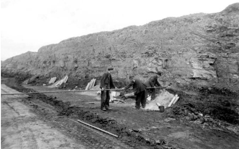
Tamping a horizontal blast hole in a sandstone above the Fenton Seam in South Yorkshire. 1945
